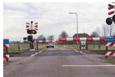
Figure 5. Mini AHB with shortened aluminium barriers and integrated led lights
