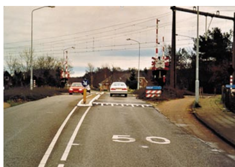
Figure 4. AHB with raised median kerb and speed bump
