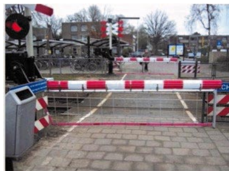
Figure 9. Barrier with skirt at pedestrian crossing in station
