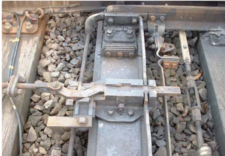
Figure 2 - Standard Facing Point Lock
